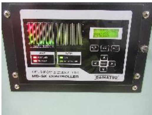
Randomly test for oil mist alarm, ok
