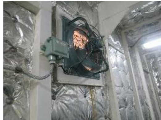
Mechanical ventilator in CO2 room operative
