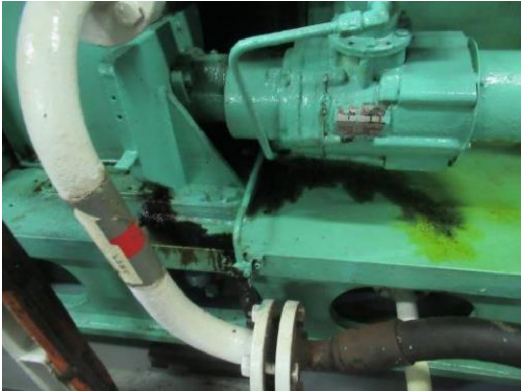
Picture 14-2: spilling oil was observed for both generator of No.2/3.
