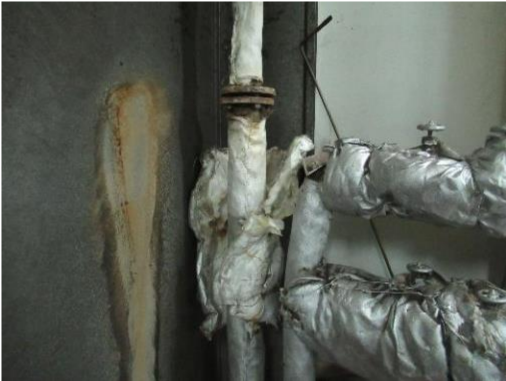
No.15 -1: Insulation laggings for hot surfaces and flanges in engine space were observed broken and oil taints.
