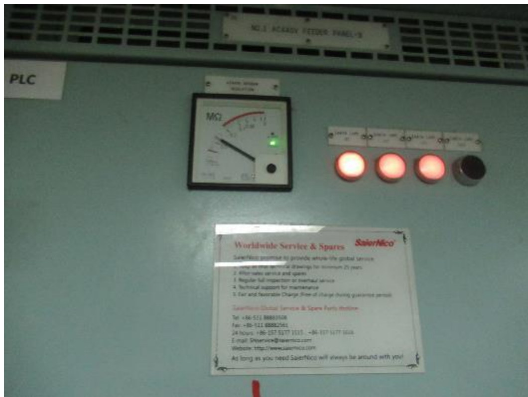
No.17 : the insulation resistance for 440V systems was found below 1 M during inspection.
