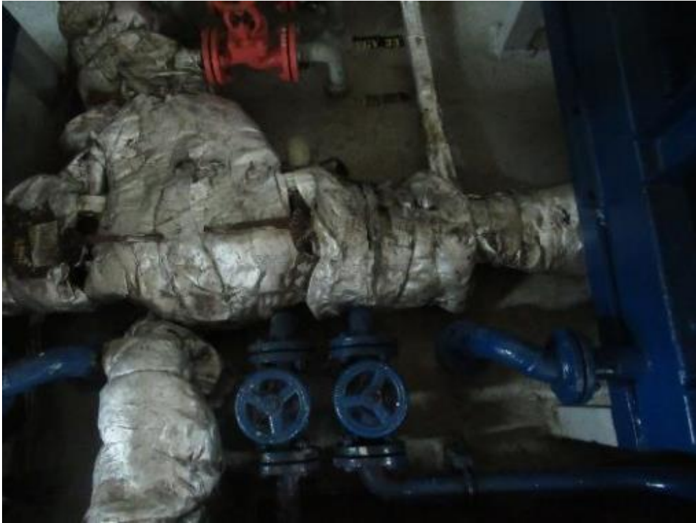
No.15-2 : oil taints and broken insulation laggings on the hot pipes in purifier were observed.
