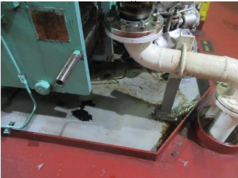
Picture 14-1: Oil leakage was observed under No.2/3 generator. Need to inspect and removal asap.
