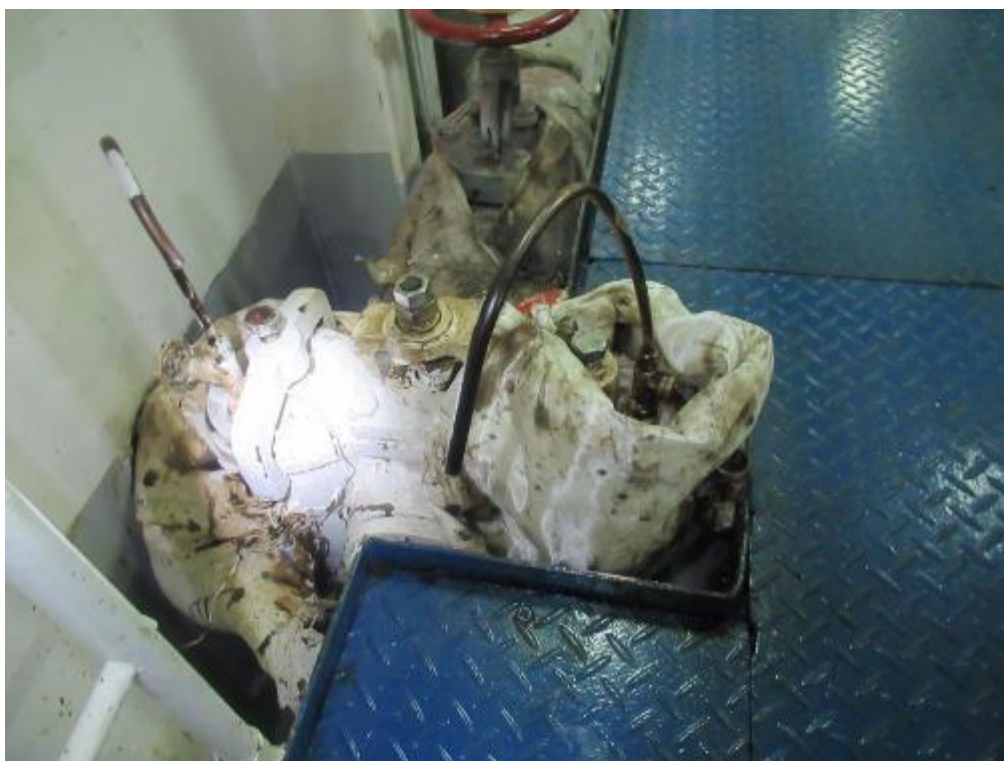
Picture 15-1: - The Purifier room was found dirty and oil leakage, black oil tant was observed on the heat insulation lagging .
