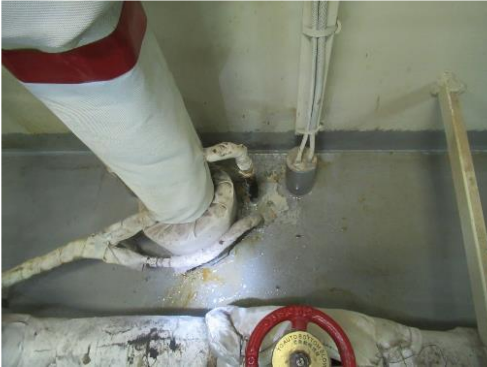
Picture 10: Continuous dropping oil from Level gauge of HSFOT was observed
