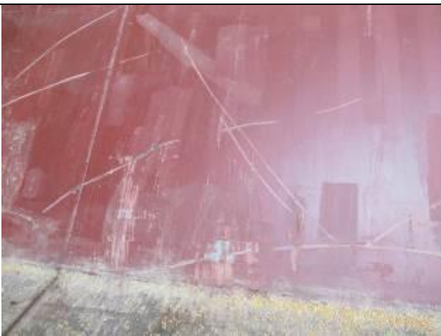
Lower hopper with lifting paint
