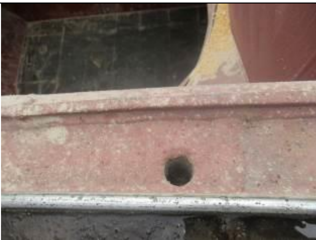
Drainage channel & drainage hole
